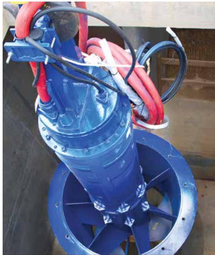
Image 1. One of five submersible propeller pumps for The Blue Plains Water Treatment Facility in Washington, D.C. (Images courtesy of KSB)
